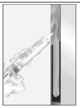
3. Gun, trowel, or pump Sonolastic NP-1\* or Sikaflex 2C or 1-A\*\* caulk to minimum 1/4" depth on both sides of wall or top of floor over the backer rod.
